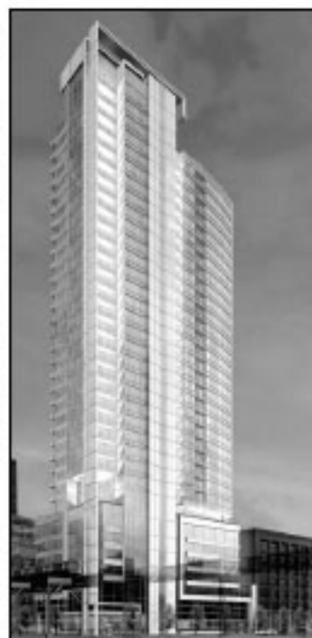
Condos start at $259,900 at Silver Tower, a 39-story high-rise planned at 303 W. Ohio.
