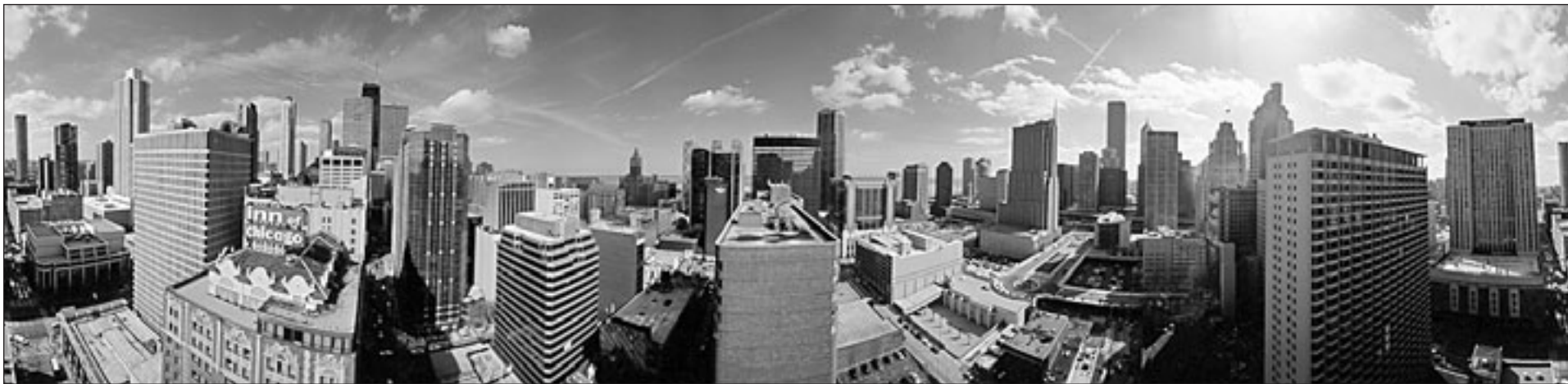
Construction is underway at 550 St. Clair, an ultra-modern 26-story condominium building in Chicago's Streeterville neighborhood. Residents will have amazing views of the city, as well as proximity to all the Chicago nightlife has to offer.
